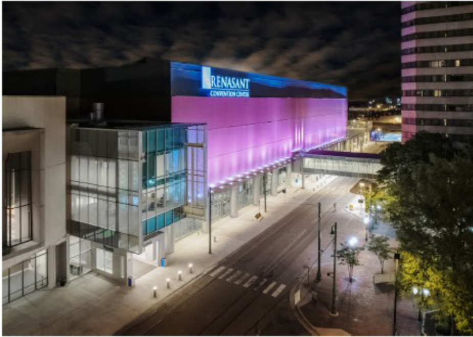
The 2026 Memphis Forum is being held at the Renasant Convention Center, which connects to the Sheraton Memphis Downtown Hotel via skybridge across Main Street. The Sheraton Memphis Downtown Hotel is the headquarters hotel. Other Forum hotel options are within walking distance to the Renasant Convention Center.
